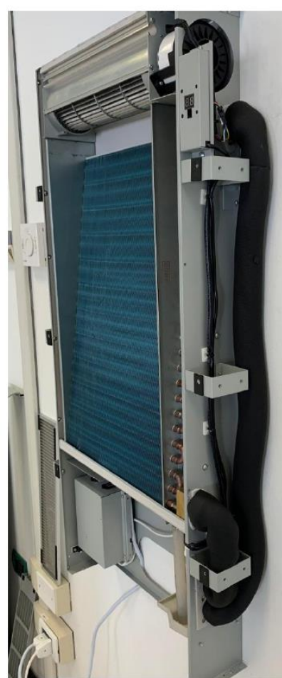
PUT INSULATION IN ALL THE EXTERNAL PIPE
