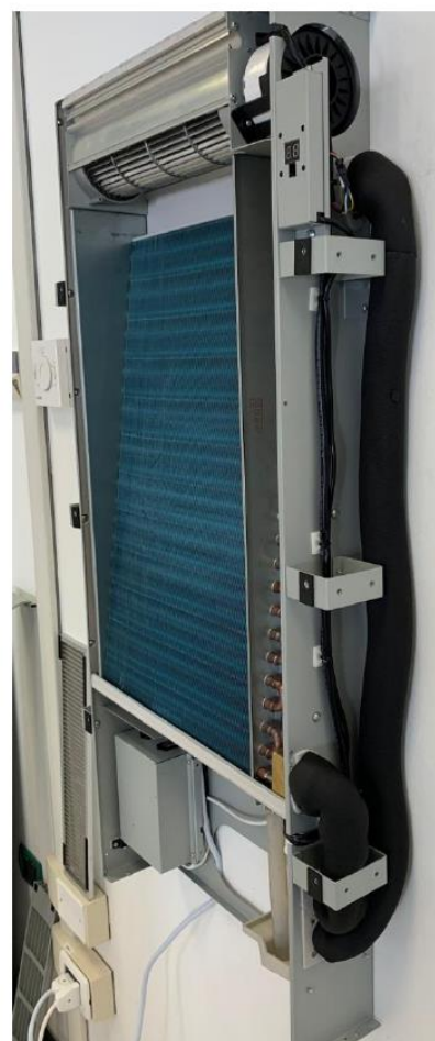
PUT INSULATION IN ALL THE EXTERNAL PIPE
